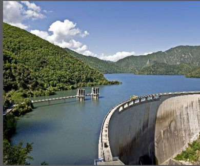
Susqueda – Spain 86 MW | 140 GWh
