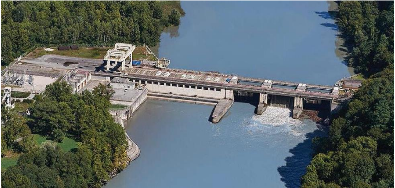
Picture 1 : Beauvoir hydro powerplant
