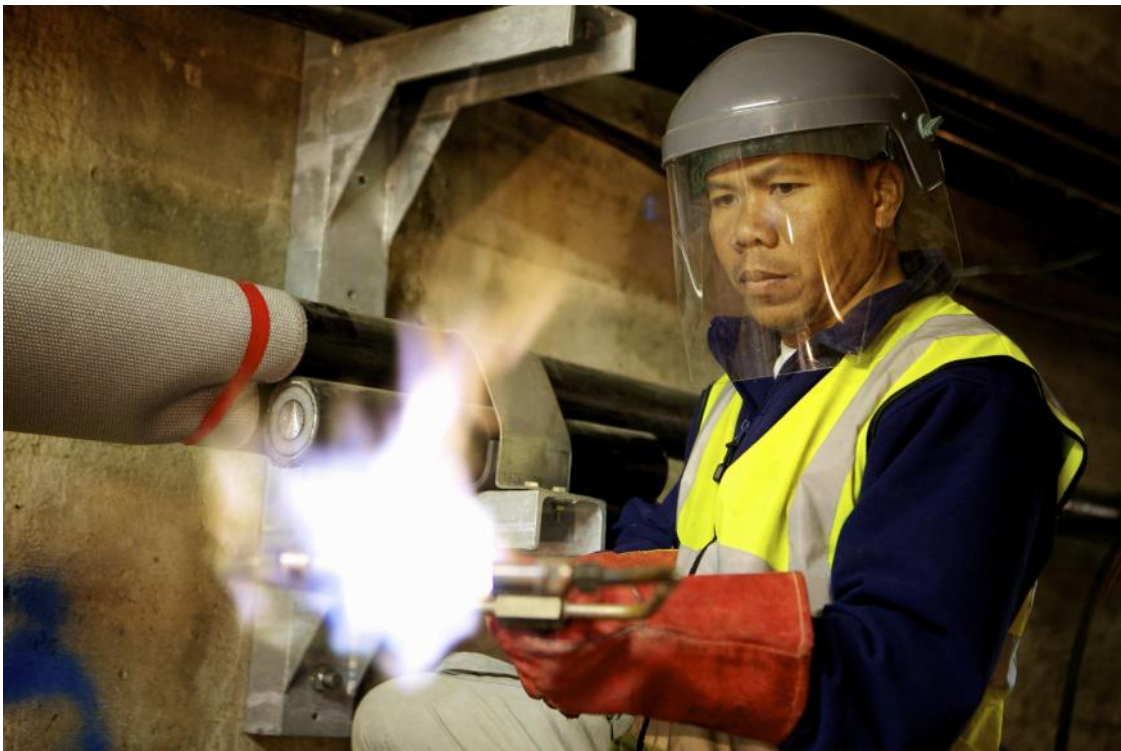
Figure 7: Construction of power distribution networks, Jersey
