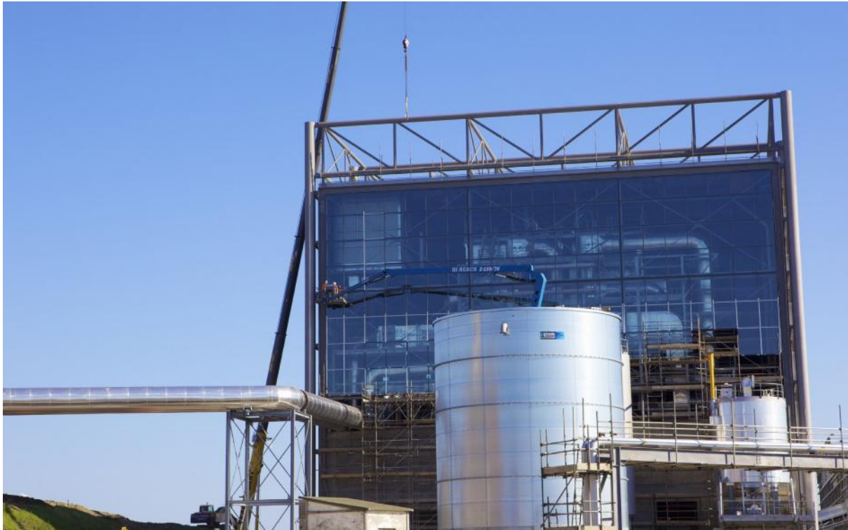
Figure 12: Construction of the 'Energy from Waste' plant, Jersey
