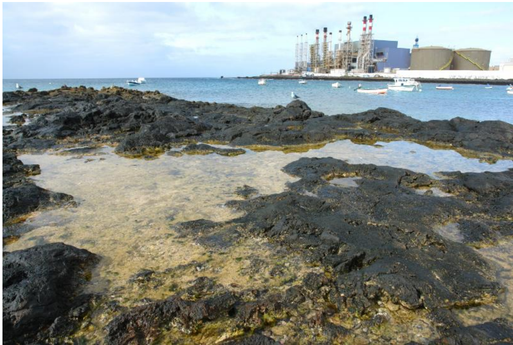
Figure 2: Punta Grande diesel power station, Canary Islands 6
